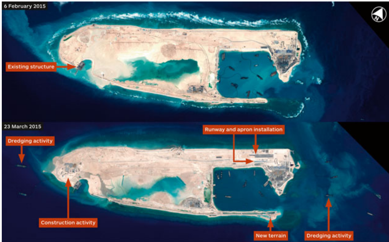
China has begun runway construction at Fiery Cross Reef in the Spratly Islands, satellite imagery dated 23 March and provided by Airbus Defence and Space shows.
