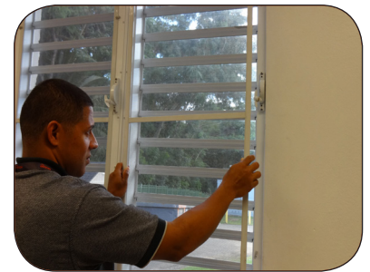
Install or repair window & door screens.
