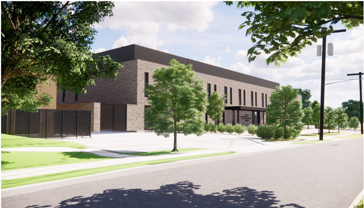
Takoma Park/Silver Spring Catherine and Isiah Leggett Math and Science Building Rendering
