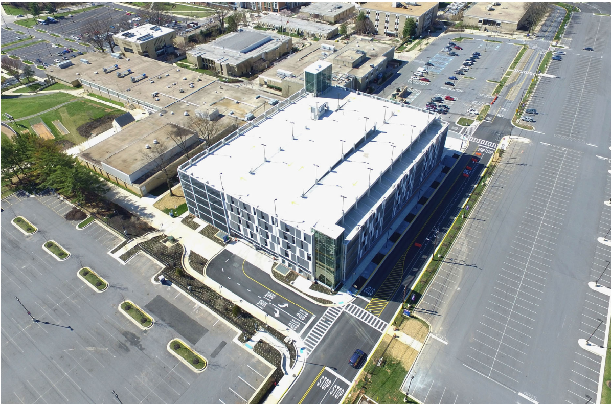
Rockville North Campus Garage
