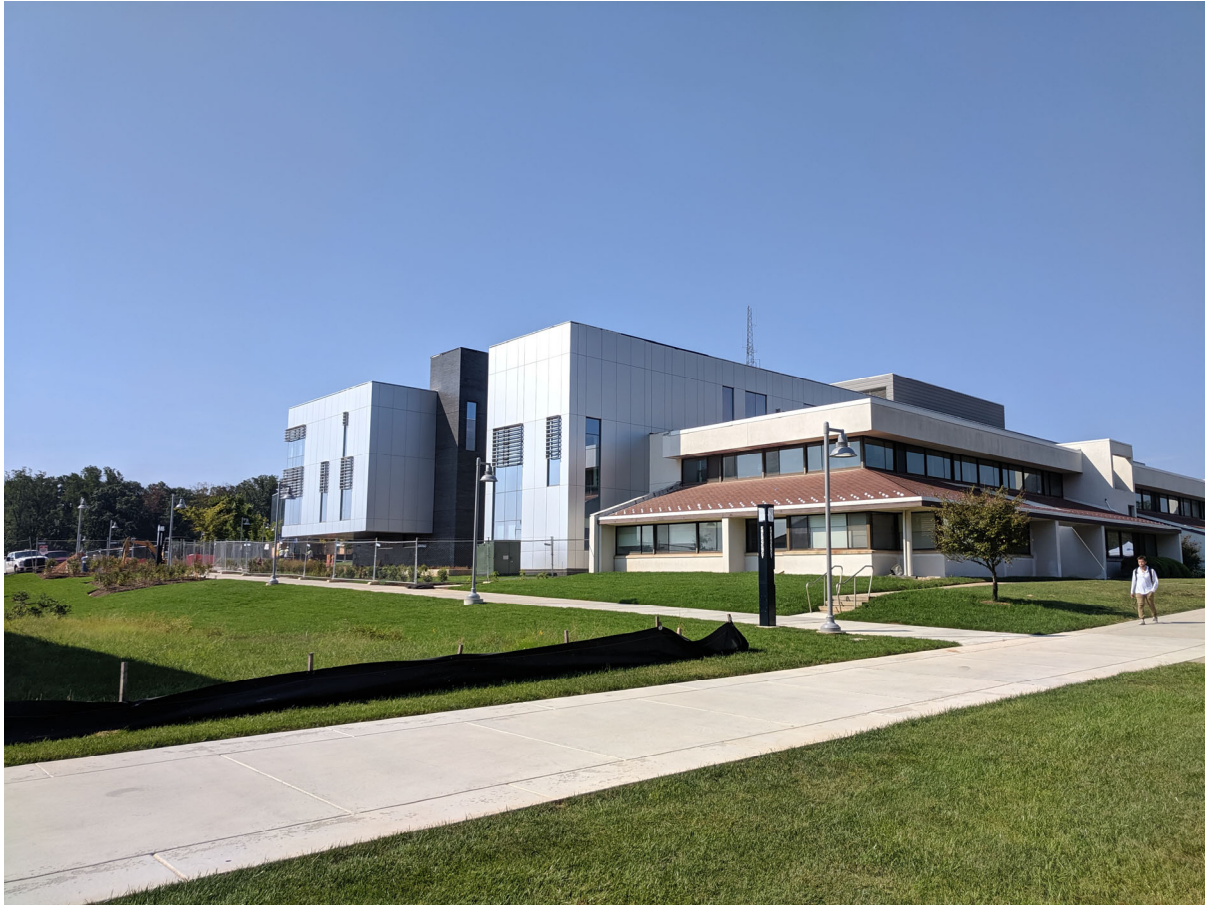
Germantown Student Affairs and Science Building Renovation and Addition
