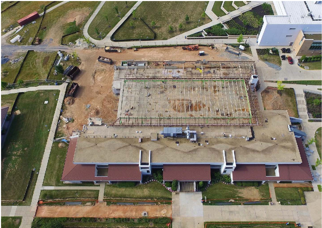
Germantown Science and Applied Studies Renovation Phase 1 as of July 2017
